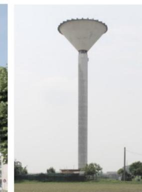
Fig. 0.3 Serbatoio "a fungo"
