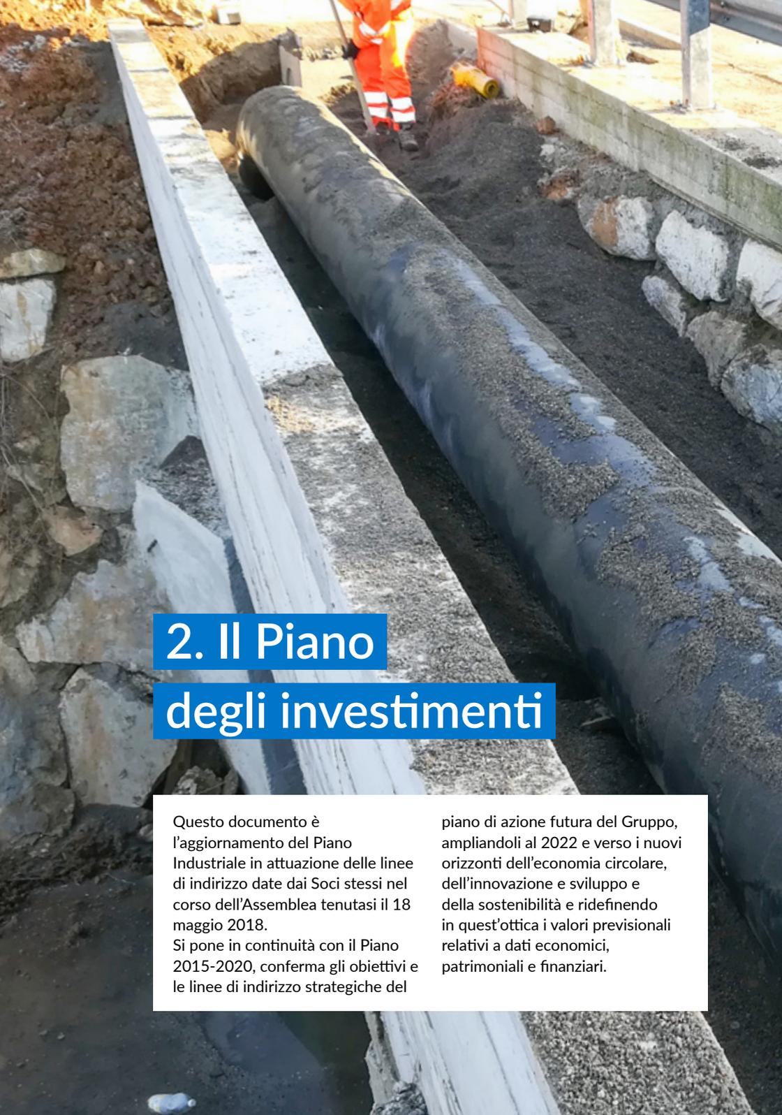
A large black pipe is being installed in a trench. The pipe is laid on a bed of gravel and is surrounded by concrete walls. A worker in an orange safety suit is visible in the background, standing near the pipe. The scene is outdoors, with sunlight casting shadows on the ground.
